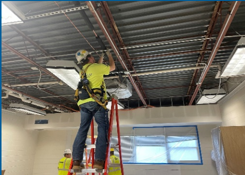
Insulation of line sets in Area D-West
