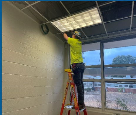
Installing low-voltage data drops in Area B
