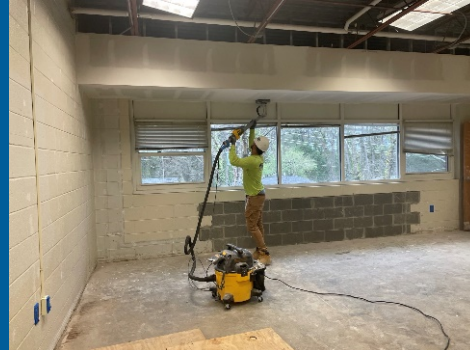
Finishing of Soffit in Area D-West
