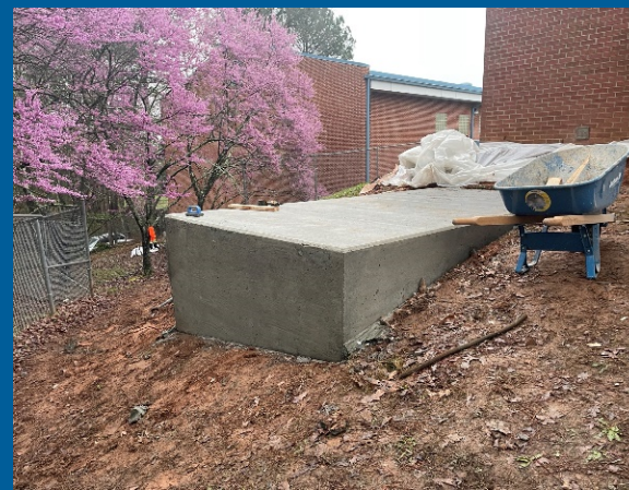
Outside Equipment Pads Poured
