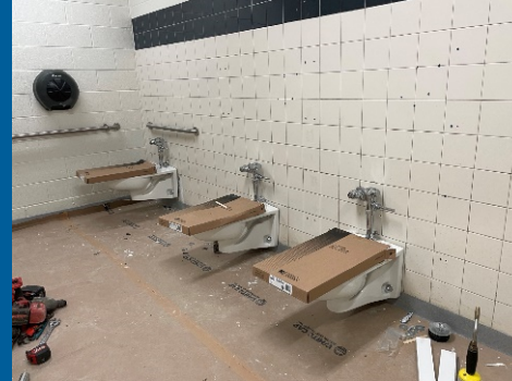
Restroom Fixtures Installed in Area A,B
