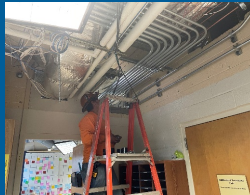
Routing Line-sets to Branch Selectors in Area E
