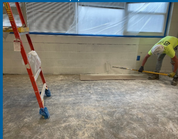
Primer Coat being applied in D-West Classrooms
